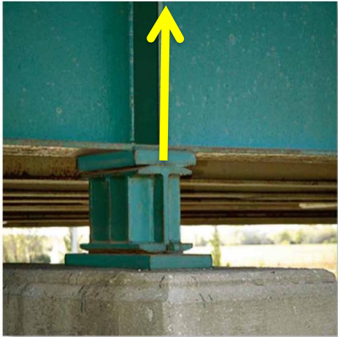
unfig05_02.jpg - The rocker support for this bridge girder allows horizontal movement so the bridge is free to expand and contract due to a change in temperature. (5) The rocker support for this bridge girder allows horizontal movement so the bridge is free to expand and contract due to a change in temperature. (5)
